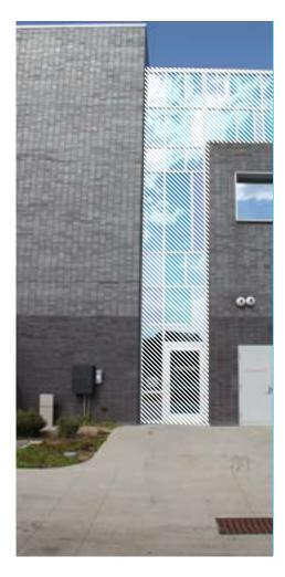
The MSU Denver HLC building accentuates a secondary entrance by providing a vertical band of glazing that extends to the roof. This change in material highlights the entry through contrast both during the day and at night.
