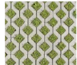
Pavers that allow for the water to permeate through what would otherwise be an impermeable surface can also provide visual interest through pattern and texture.
