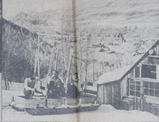
THE BOAT TOW already installed on the Roch run loads skiers halfway up the practice hill, where they are brought by a rope tow, and takes them 550 vertical feet to the top of the 1600-foot long practice slope. Three skiers are shown with their skis loaded on the racks, the high-altitude sun full upon them, set for the trip to the top. The girl in front is Virginia Heidecooper, one-time woman's national champion skier. The girl in the back is the author.
